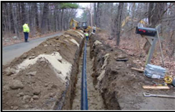
Water main installation along Haynes Rd. to provide water to new Patriots Common Development
