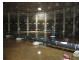
The Tideflex Mixing System installed
