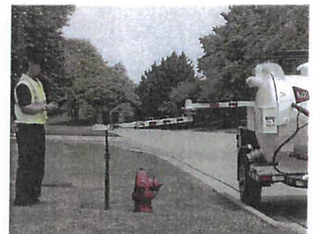
ERV-750 extended reach valve exerciser allows valve operation from the road, removing the need to pull onto the grass
